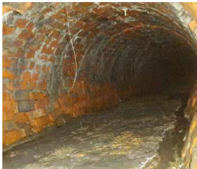
During the Winckley Square restoration work in 2016 the original pre-Victorian culvert was reinforced and linked with modern drainage systems to reduce seasonal flooding of the site.
