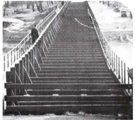
Tram Bridge minus timber decking 1946 which had been removed for the duration of the war to block any German advance. Harris Museum, Art Gallery and Library.
