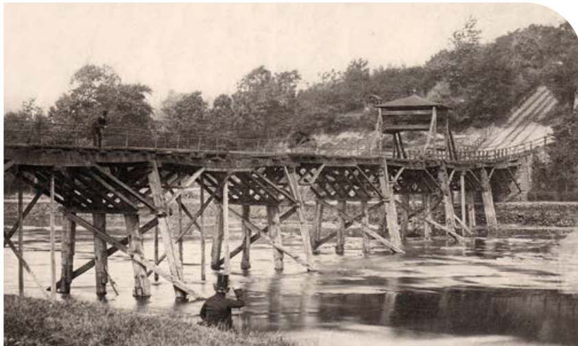
The Tram Bridge c 1864: Robert Pateson, Preston Digital Archive. The chain ran between the housing drum on the bridge to the upper drum located to the left of the Engine House at the top of the incline.
